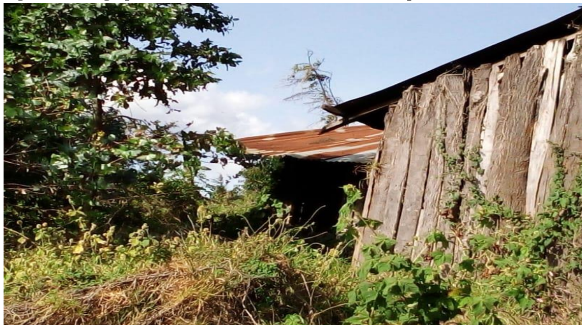
Figure 4: Photographs of some of the vacated homes due to the perennial clashes
