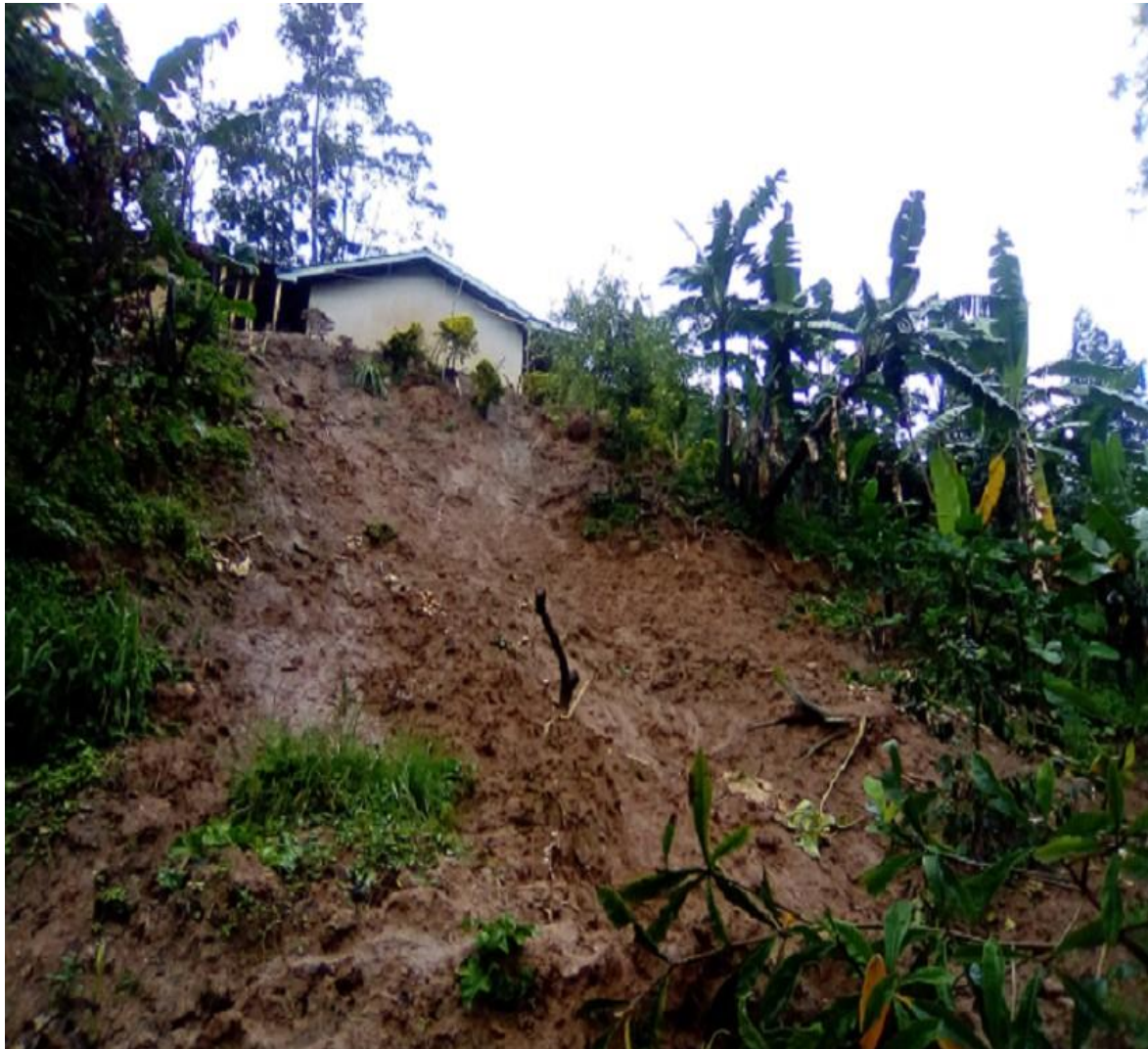
Figure 12: A landslide very close to a home in Bundesi Parish. Photo taken by Mande, November 2020
