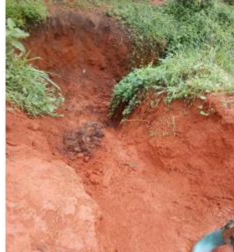
b) Trench damaged by elephants
