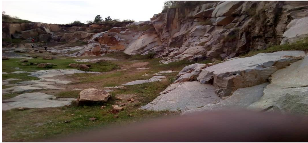
Plate 3: part of the quarry site in Petta where 2 people were buried by collapsing cave in 2020
