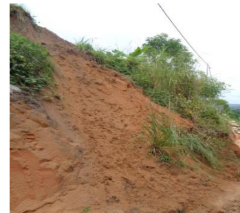
Figure 22: Landslide of Gully Walls Along the Road Shows Evidence of Undermining at the Base and/or the Presence of Clay.
