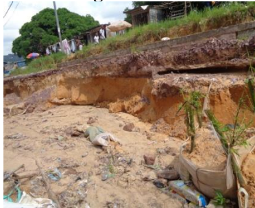
Figure 18: Km5: Failure of the Work Initiated by a Chinese Company Responsible for Resurfacing the Road.
