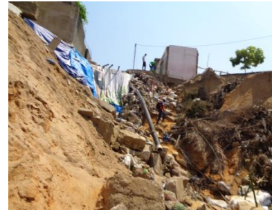
Figure 22: Landslide of Gully Walls Along the Road Shows Evidence of Undermining at the Base and/or the Presence of Clay.
