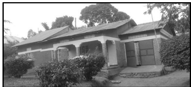
Figure 3: Garage room for a car transformed into a rental space
