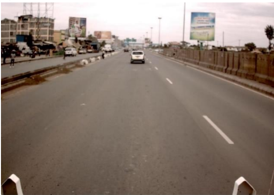
Figure 3: Pavement surface condition
