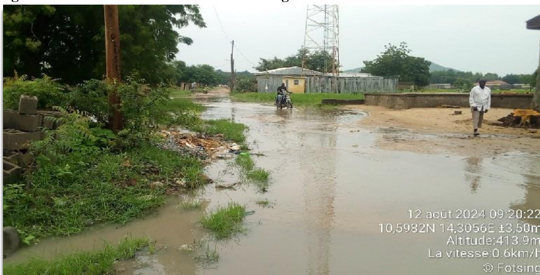
Figure 18: Obstruction of Rainwater Drainage Channels in the Pitoiré District
